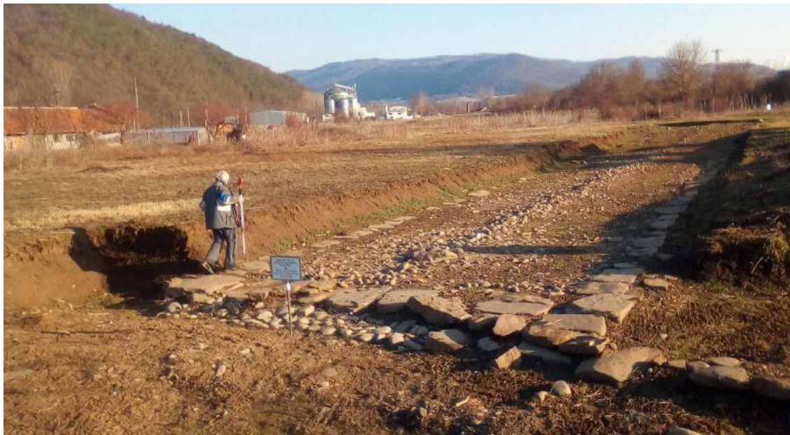
Figure 11 Part of Via Traiani right in front of the Sostra castellum (authors' archive)
